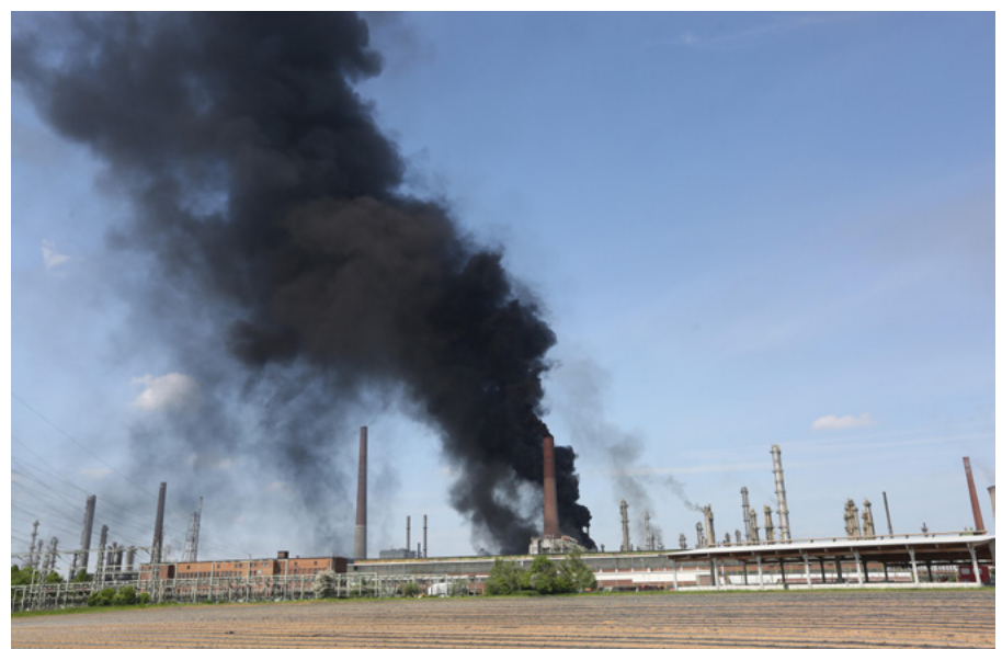
Shell Refinery Wesseling
